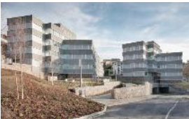
41. Beldarrain Studio / Housing for young and elderly people, Donostia, País Vasco, Spain, 2008
