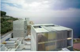
44. MGM Arquitectos / Housing Monte Hacho, Ceuta, Spain 2009
